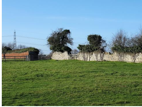
Walls of Cotes Old Hall as viewed from the footpath H96
